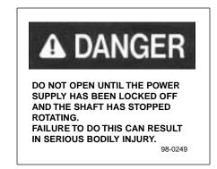
The above DANGER decal is placed on all **nyb** cleanout doors. These doors, as well as access doors to the duct system, should never be opened while the fan is in operation. Serious injury could result from the effects of air pressure or suction.
